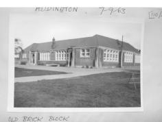
Figure 19. Addington School: Penlington's original building, modified by the removal of gables and the introduction of a hipped roof in an attempt to secure the structure against possible earthquake damage. Reference: CEB Building Ledger, ANZC, CAMQ, 12457, CH437, box 2, 110d.
