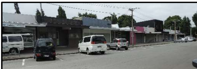
12 shops in Acheson Avenue Shopping block. A Dairy open to community, remaining used as business storage, residential unit or vacant. Unmaintained and untidy appearance.
