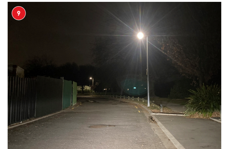
Glare created by led lighting in the laneway.
