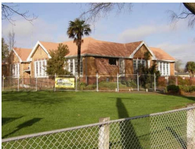
Figure 1: The former Shirley Community Centre, shown here post-earthquakes
